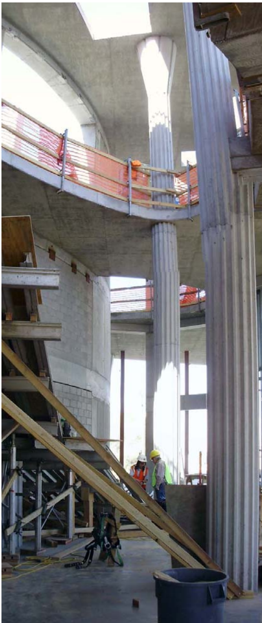
Center for the Arts lobby under construction
