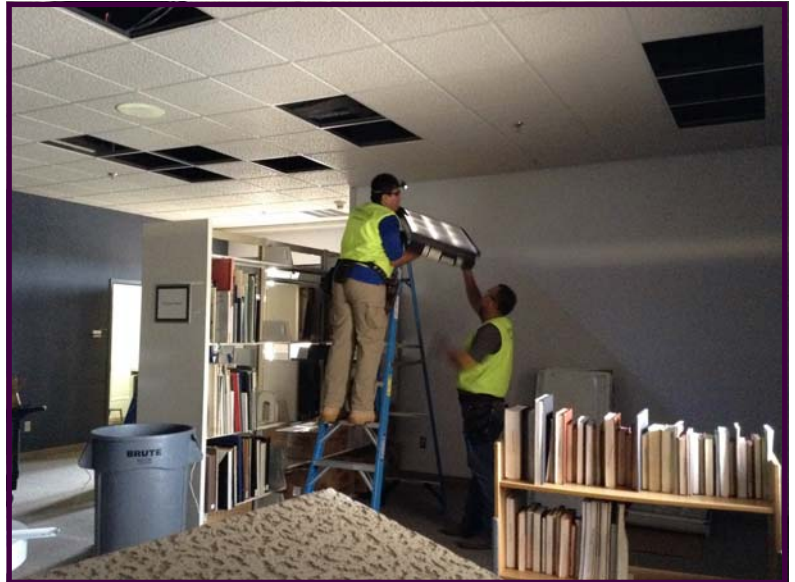
Instead of retrofitting, installing entirely new fixtures in Zuhl Library stacks
