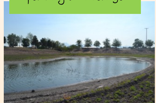
Water retention pond at Sam Steele Way Dr. and Union
