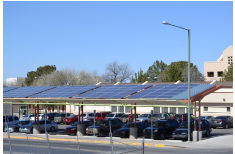
Solar panels outside the Campus Health Center provide approximately 25% of the energy needed for the building as well as provide shade for the parking lot.
