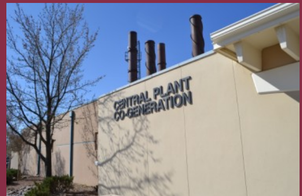
The Central Utility Plant is where campus utilities are managed
