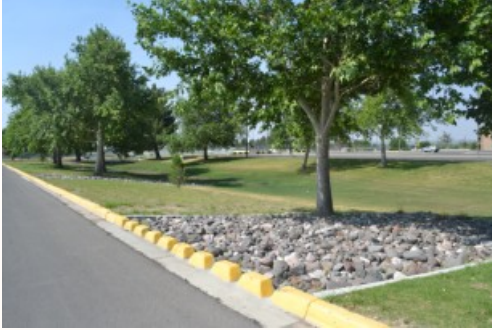
This is an example of stormwater management to the west of Pan American Center
